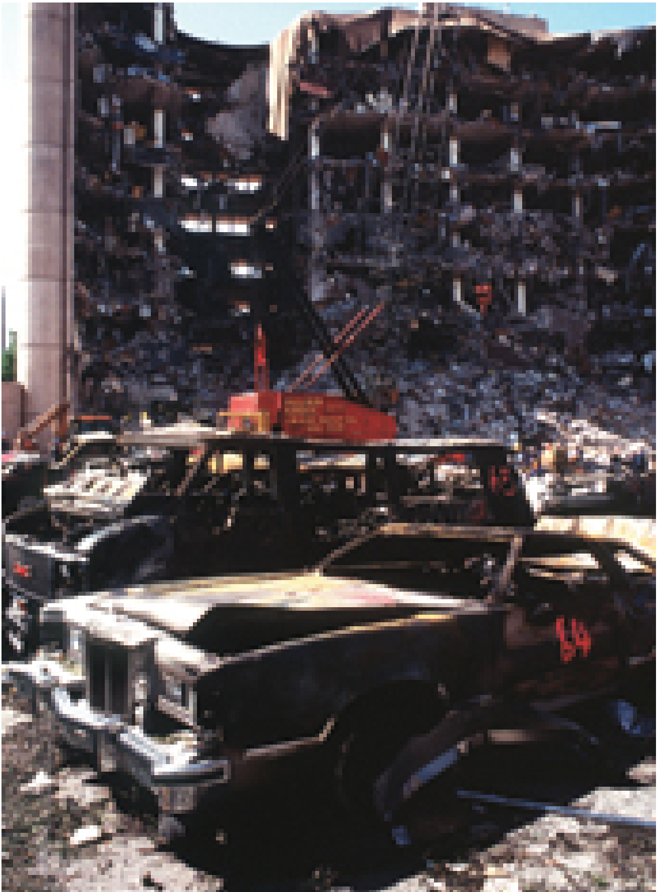
Alfred P. Murrah Federal Building, Oklahoma City.
